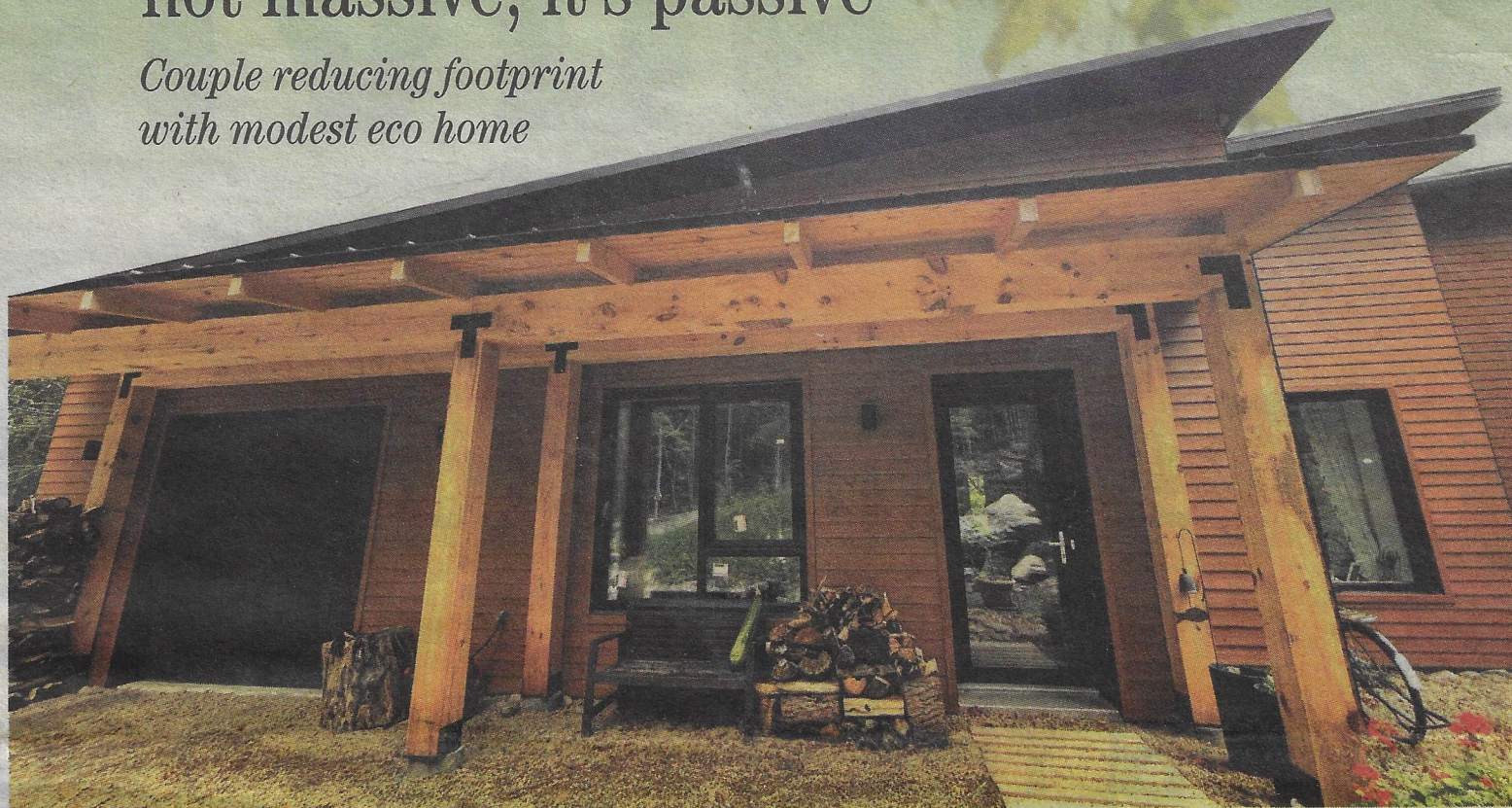
This passive home in Chelsea was designed by EkoBuilt and constructed by Wakefield builder Marilyse Bisson of Mavie Construction. The modest, 1,700 square-foot home, including a garage, boasts triple-pane floor-to-ceiling windows, 15-foot ceilings and a high-efficiency wood stove. Trevor Greenway photo
